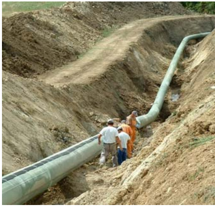
Figure 9: SMARTape on the gas pipeline.
